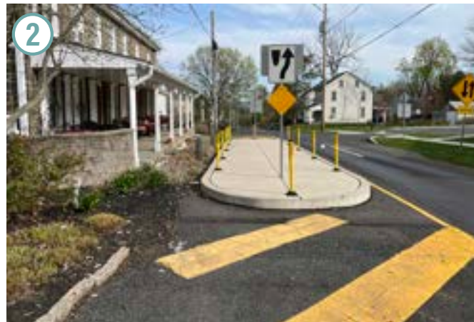
2 Traffic barrier installed on Old Skippack Road
