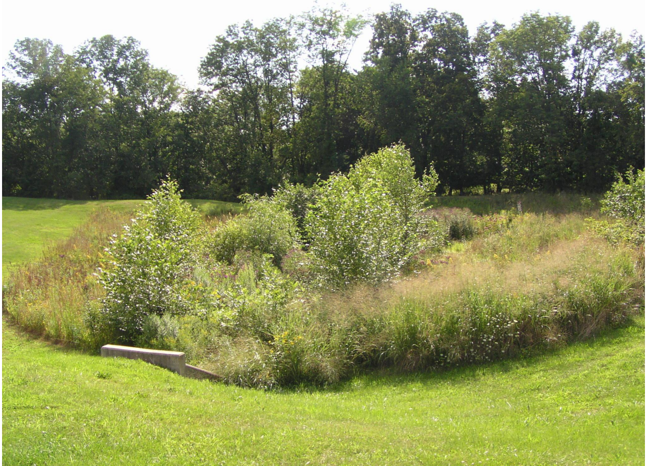
A stormwater basin filled with native flowers, shrubs and trees in Upper Providence.
